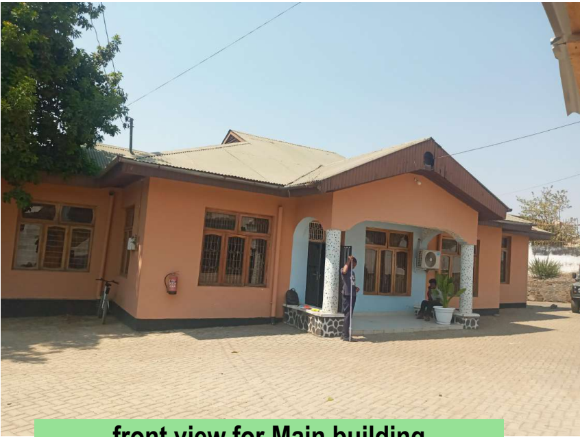
front view for Main building
