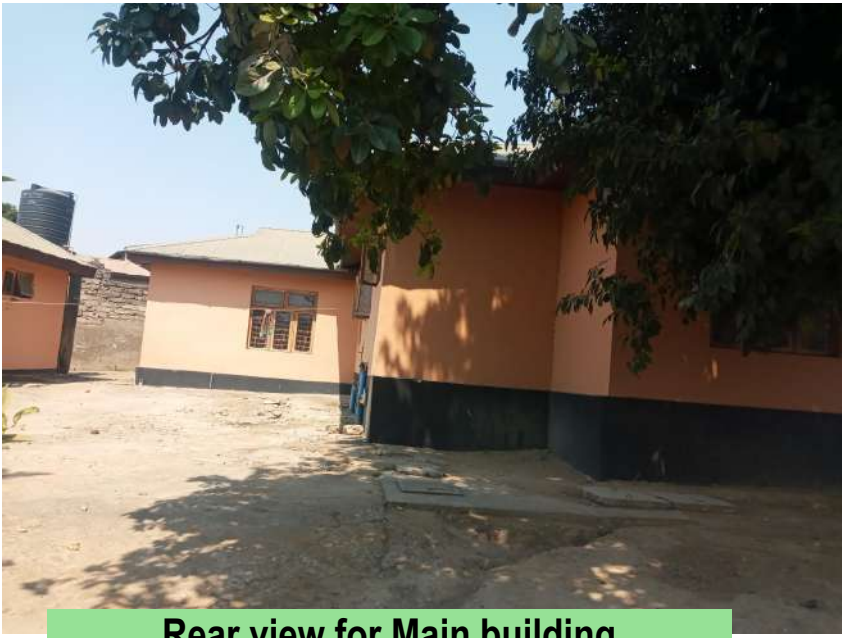
Rear view for Main building
